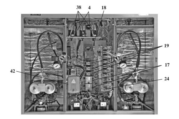
Figure 6 Model 7200 Air Dryer ( inside top view )
